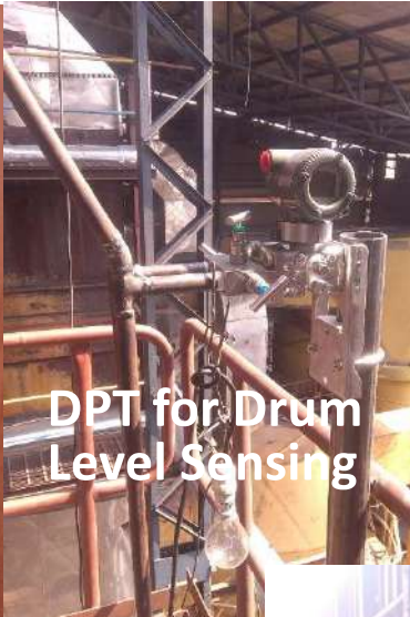
Impulse Tubing and Condensing Pots for Drum Level Sensing
