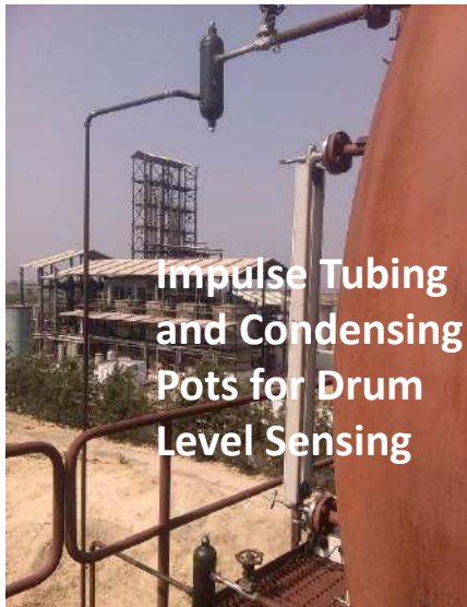
DPT for Drum Level Sensing
