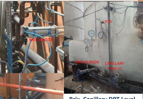
Brix, Capillary DPT Level, and RTD Temperature Sensor installed on Batch Type Vacuum Pan
